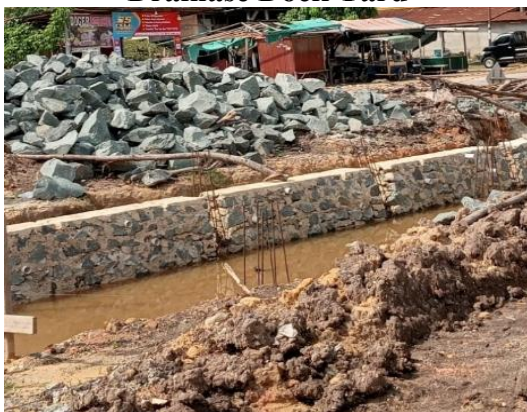
Gambar 6. Normalisasi Saluran Drainase Dock Yard
